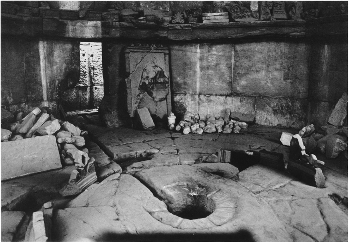
FIG. 13. Interior of octagonal tower with doorway to cylindrical water tower at left
