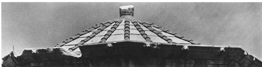
FIG. 12. Roof finial and marble roof slabs
